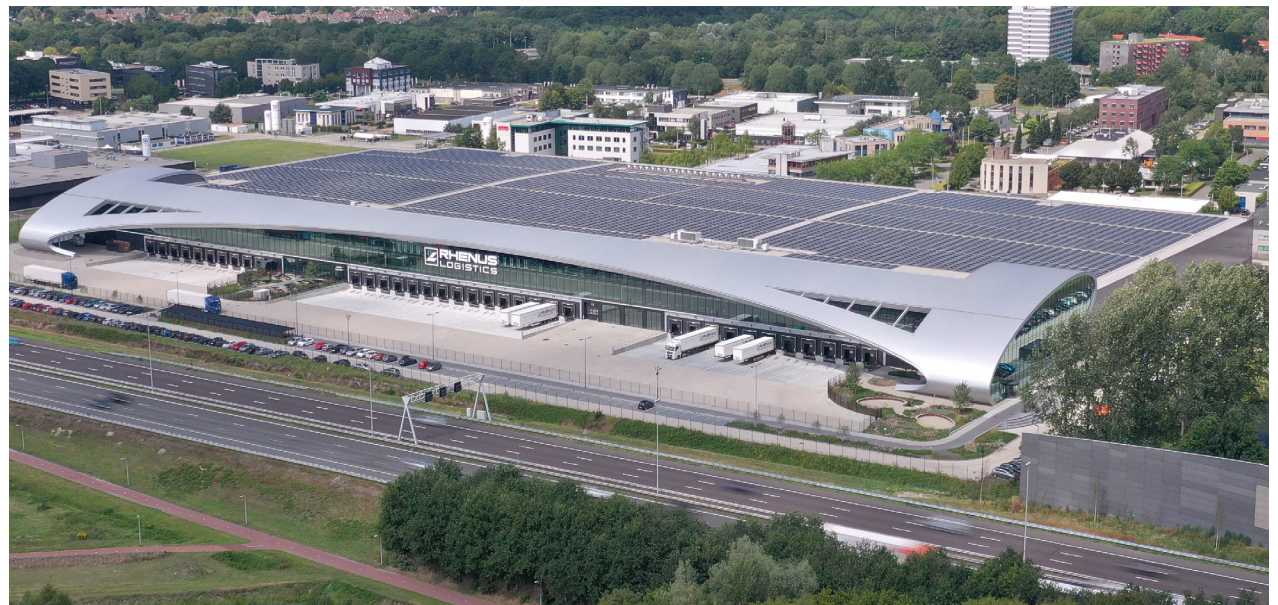
Rhenus Logistics warehouse in Tilburg, Netherlands, fitted with its own renewable power generator
