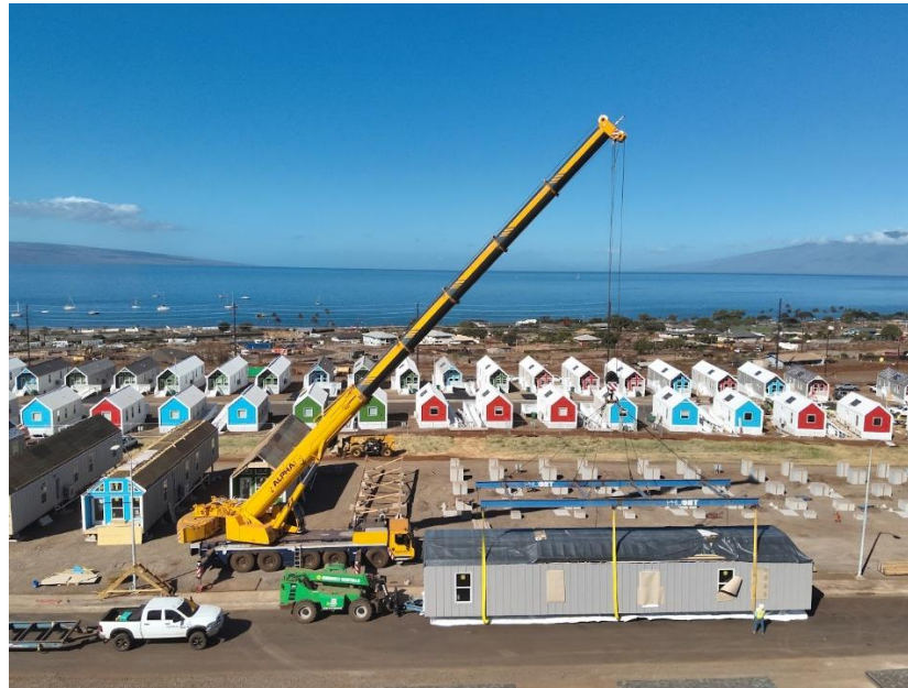
Figure 9: Homes being installed onsite at Kilohana site
