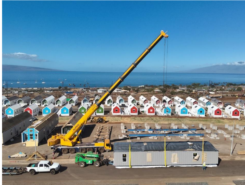
Figure 9: Homes being installed onsite at Kilohana site
