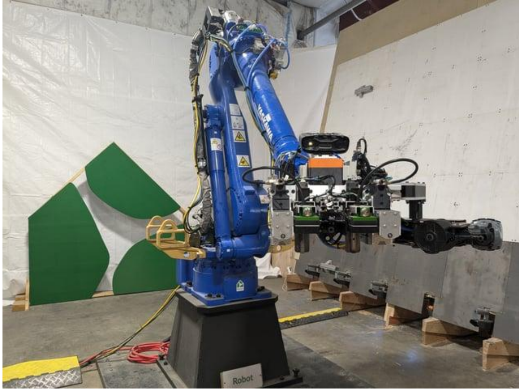
Figure 12: Robotic arm assembling a wall panel in the upright position at Reframe’s Massachusetts pilot microfactory. Source: Authors, photograph taken 2025.
